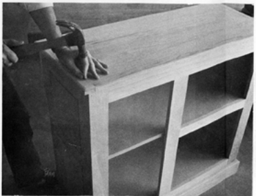
10. ATTACH TOP (U), BASE (S,T), AND TRIM (W,X) WITH GLUE AND FINISH NAILS. ROUT BACK OF UNIT FOR INSERTION OF 1/8" PLYWOOD (R). (SEE SECTION BB AND CC.)
